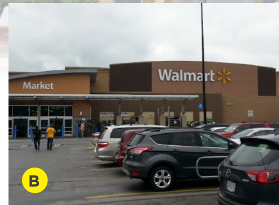
The commercial retail area just west of SOM Center Rd is a highly visited shopping area with large setbacks and parking lots.
