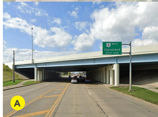
A The Route 2 underpass has existing sidewalks, but is poorly lit and creates a perceived barrier along Vine St, especially to pedestrians.
