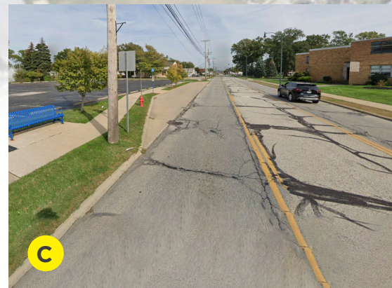
C The City of Willowick has the narrowest typical section of the Vine Street Corridor with one driving lane in each direction and one center turn lane.
